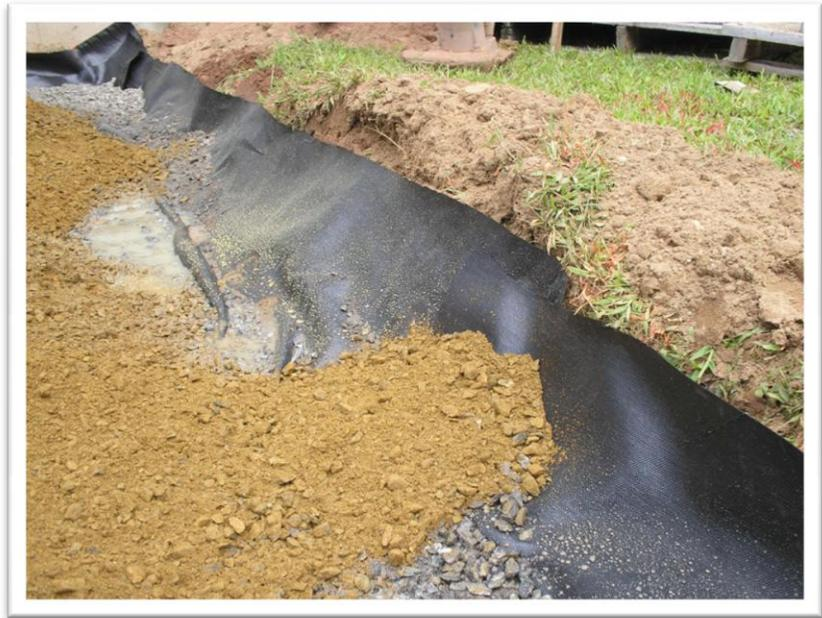
So you ask, why do I need it in my project? **LONGEVITY.** Again the ICPI states: *When geotextiles are used they preserve the load bearing capacity of the base over a greater length of time than pavement without them.*
