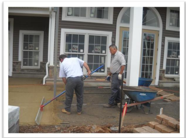
It is imperative to use the correct materials or shifting and settling could occur. Again, never use stone dust to fill the joints. It breaks down during the compaction process.
