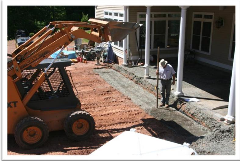
We are certainly much colder here in CT than a lot of other places in the world. Therefore, it is imperative that the base material be deeper than the recommended 4". In CT, we recommend that a paver project being completed on good, well-drained soils have at least 7"-10" of base material.
